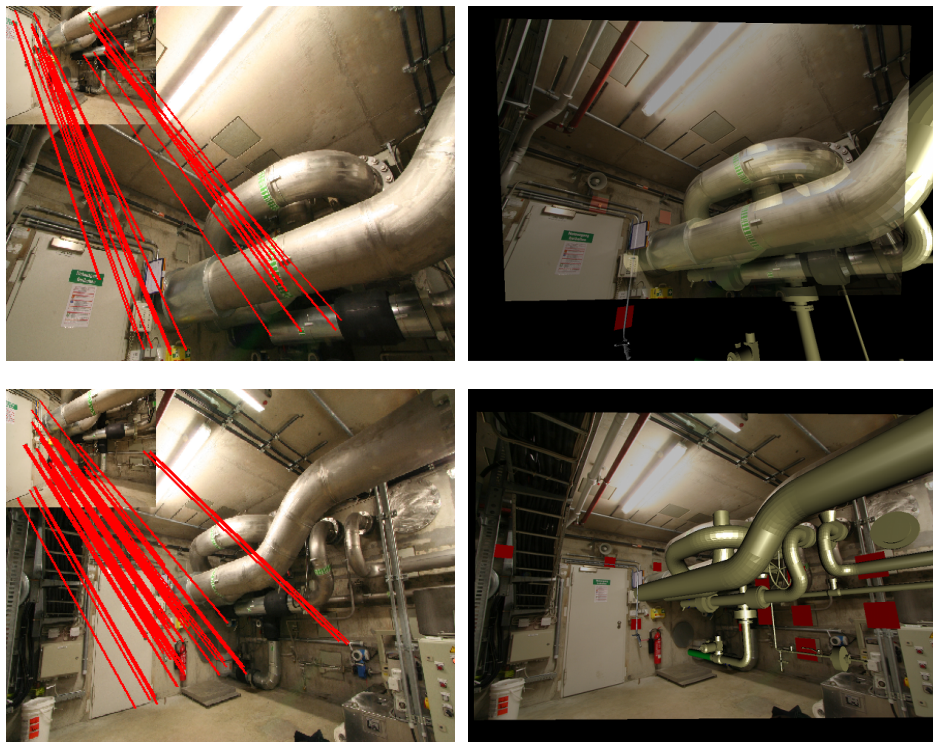
Figure 5: Real experiments: the left hand graphics represents the corresponding pair of points corrected using our method, the upper snapshot is the original keyframe; the right hand images display the resulting augmentation displayed in a VRML viewer.
