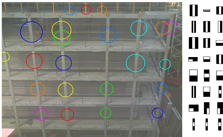
Figure 2: Example output for column detection ( left ), with Haar features used ( right ).
